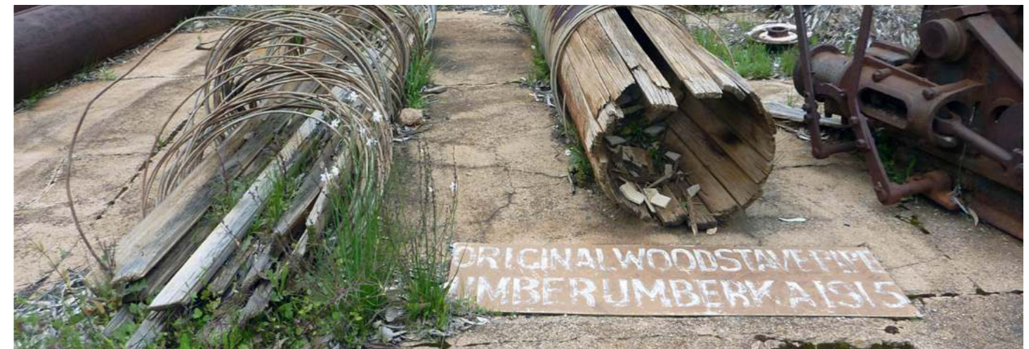
Photo: Original wood stave pipes used for gravity delivery of water from Blue Anchor Hill to Broken Hill. On display at Umberumberka Waterworks
